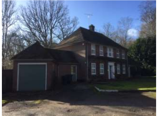
Vicarage - front view
